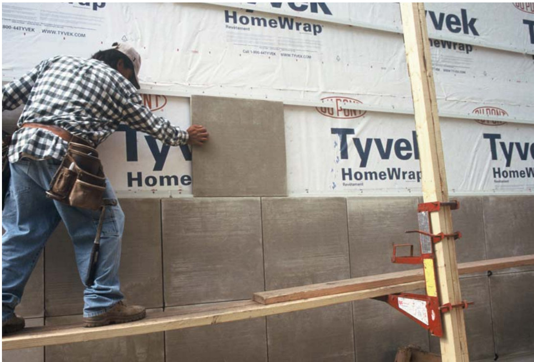
Continuous Anchor Installation (See p. 3.1.5 of ALC Solution Manual)
