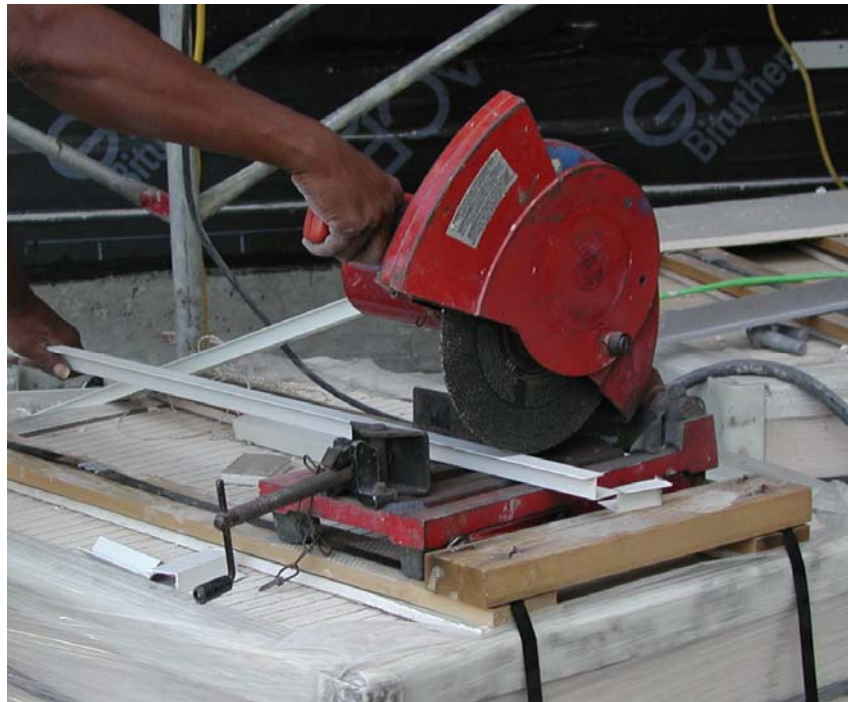
T-Anchor being cut to size on jobsite
