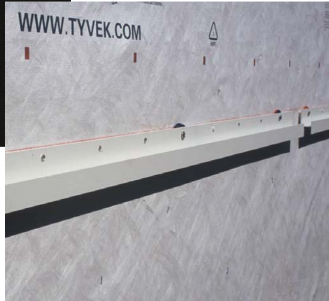
T-Anchor (See p. 3.1.1 of ALC Solution Manual)
