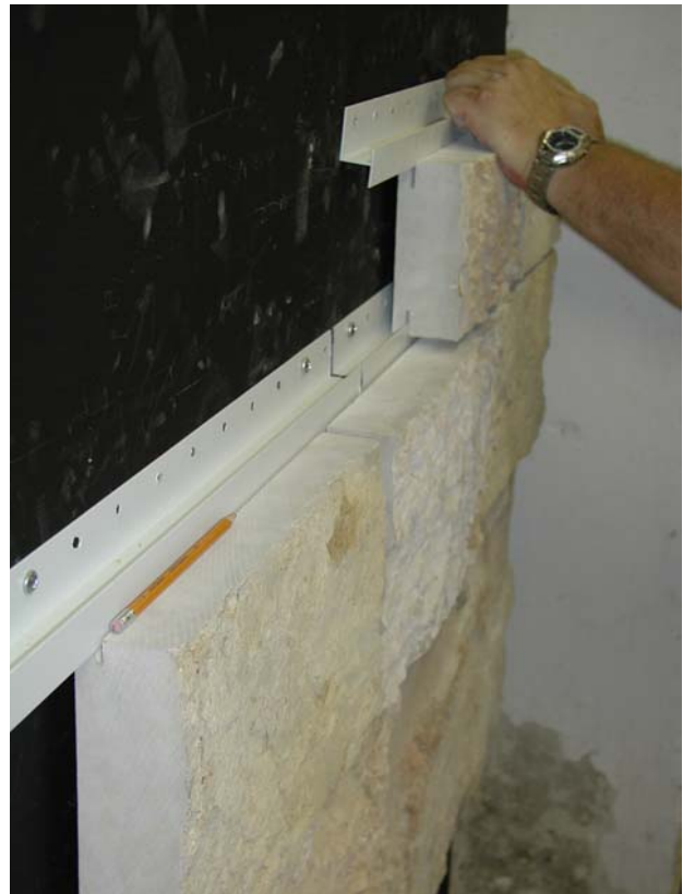
Installation of 2-Inch Thick Panels (See p. 2.6.10, 3.1.4 & 3.1.5 of ALC Solution Manual)
