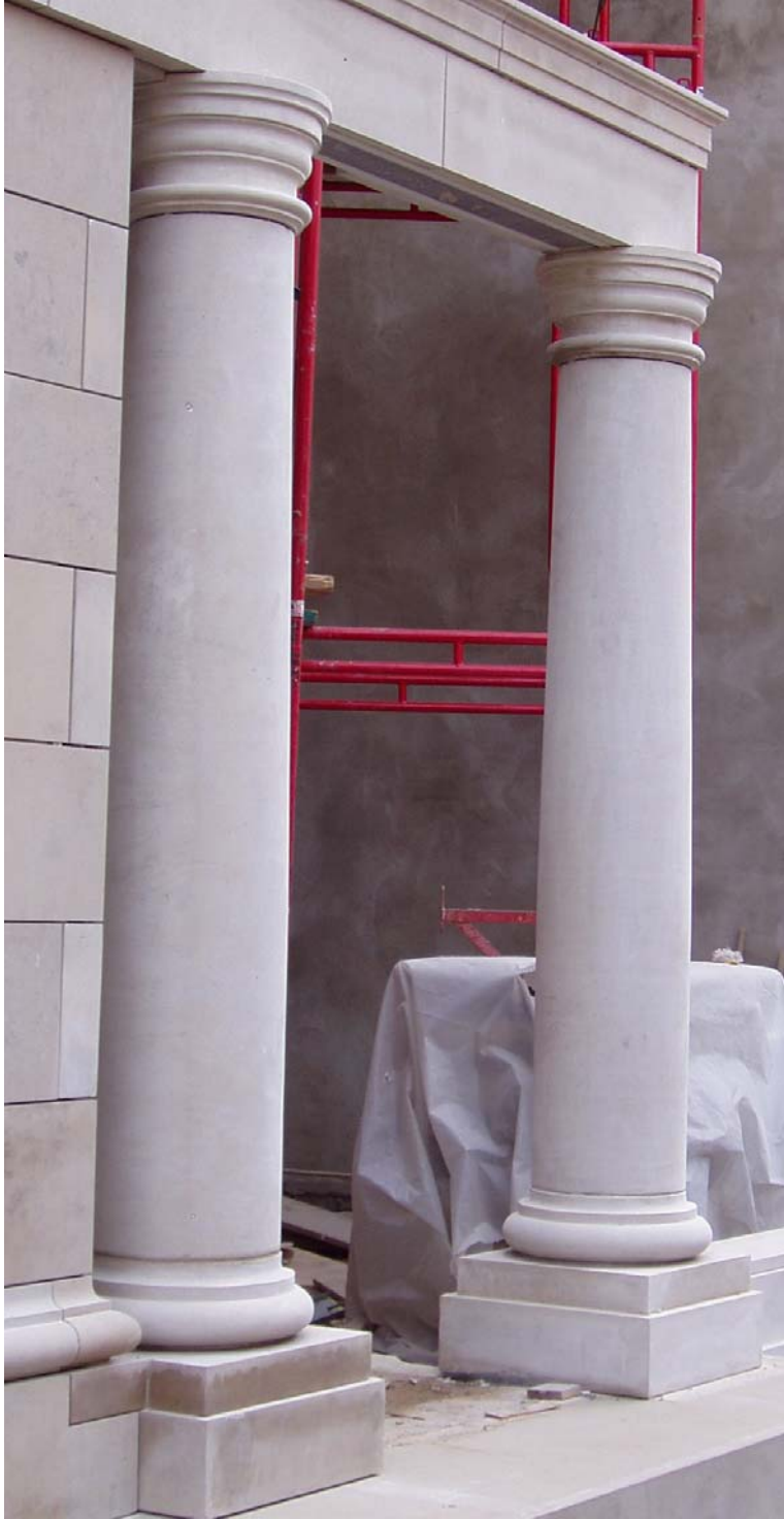
Tuscan Column (See p.1.1.5A of ALC Solution Manual)
