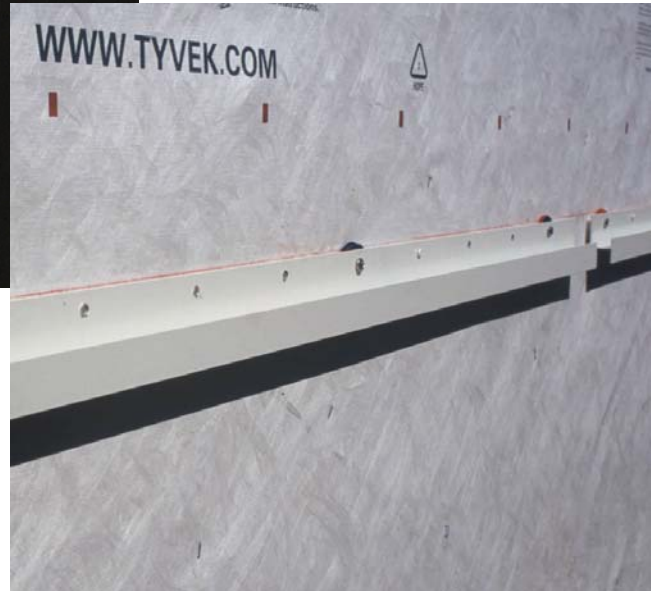
T-Anchor (See p. 3.1.1 of ALC Solution Manual)
